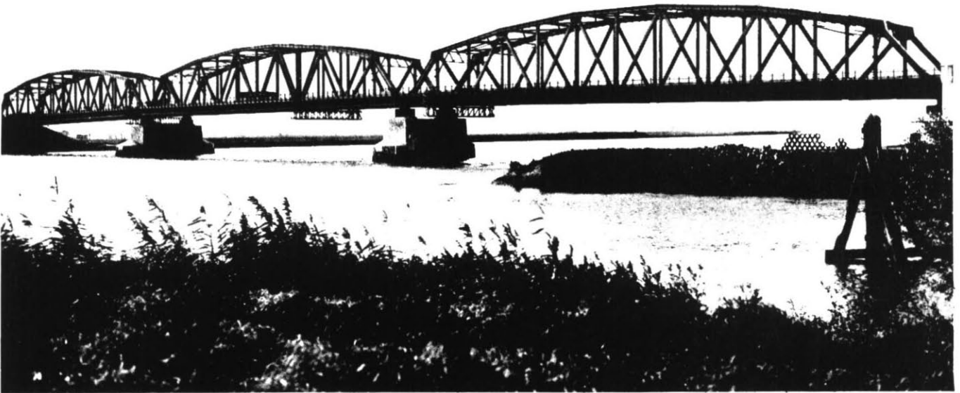
The old road bridge at Keizersveer was a trussed arch bridge. Now, this bridge has been replaced by sections of the Moerdijk bridge (see Reading Text 3).
