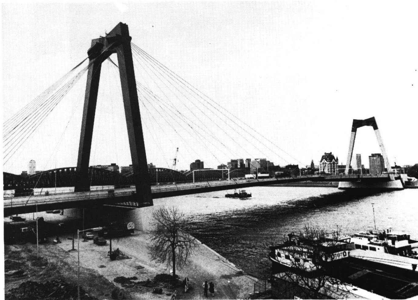
The new Willems bridge over the river Maas in Rotterdam, just before it was opened in 1981. It is a stayed girder bridge with a steel bridge-deck suspended from the A-shaped pylons.
