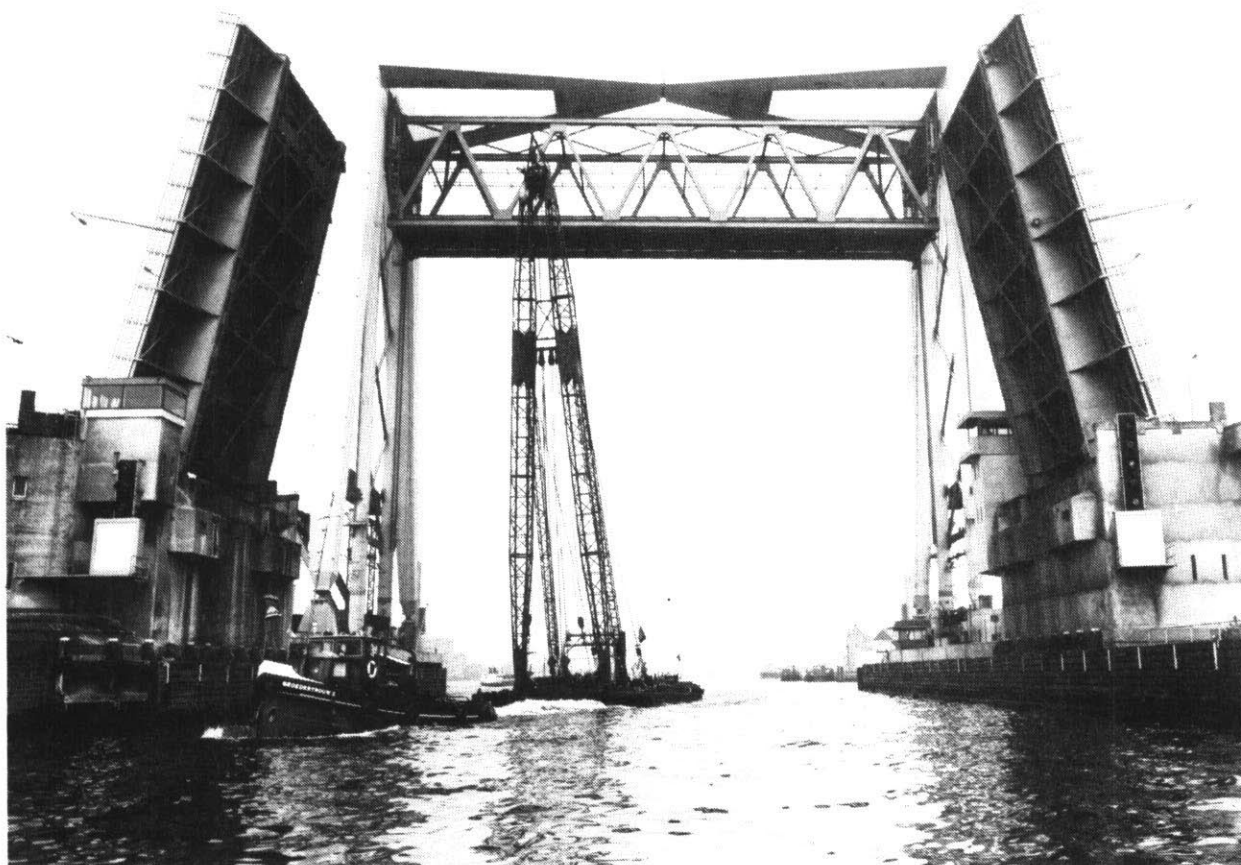
This photograph shows some of the things discussed in this theme: different types of bridges (a double bascule bridge and a lifting bridge) and a big floating derrick crane by a tug-boat. The photograph was taken in Dordrecht.
