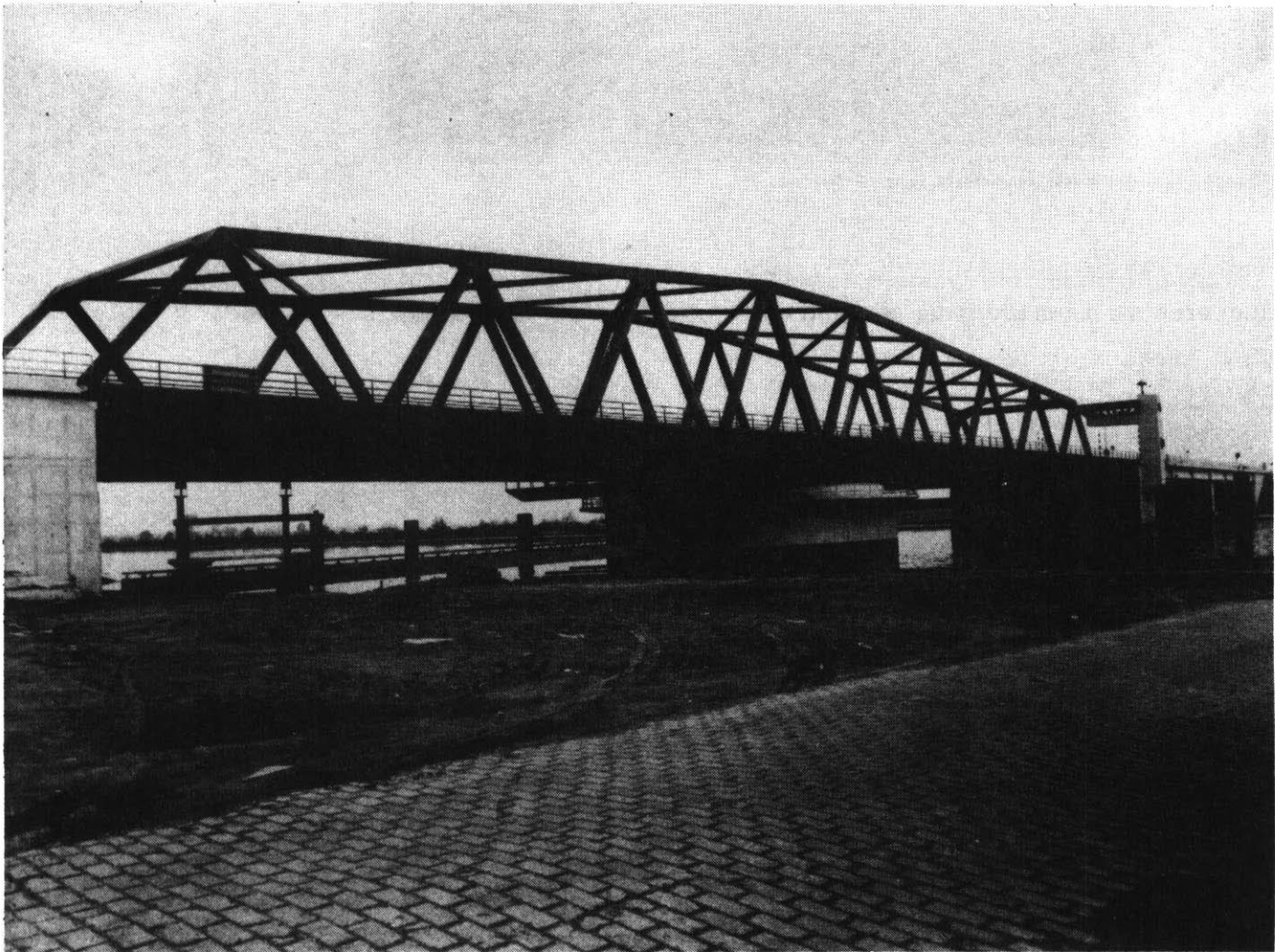
This truss bridge near Sluiskil rotates round the central pier
