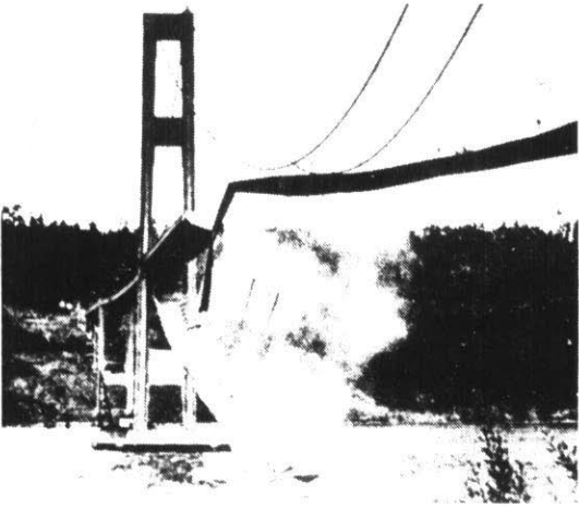
On 7th November 1940, during a gale, the new Tacoma Bridge in the United States collapsed. It could not withstand the enormous stresses.
