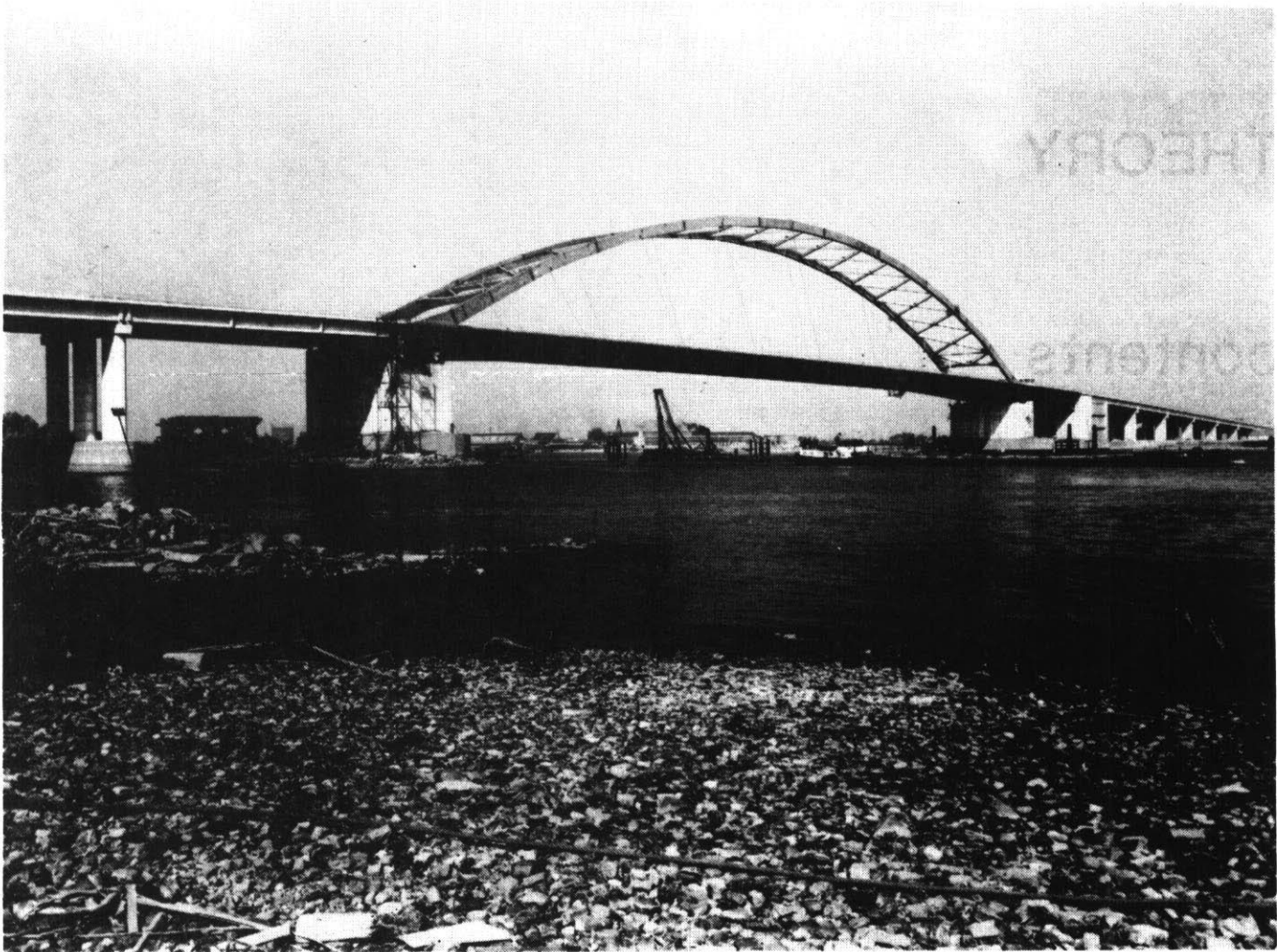
The Van Brienenoordbrug in Rotterdam has the longest span in the Netherlands: 287 m. The arch transfers the stresses in the bridge-deck to the piers.
