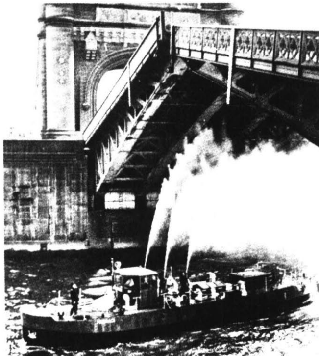
Tower bridge in London during a heatwave. The bridge-deck had expanded so much that the bridge couldn't be closed. It was cooled by water from the river.
