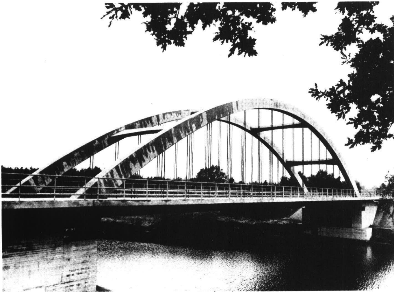
The Twente-canal bridge. The bridge-deck is suspended from the arch. Notice how the arch is supported by the piers.
