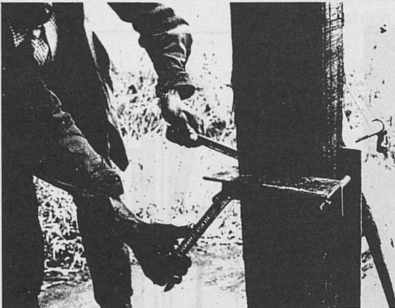
After a while the bolts must be tightened.
