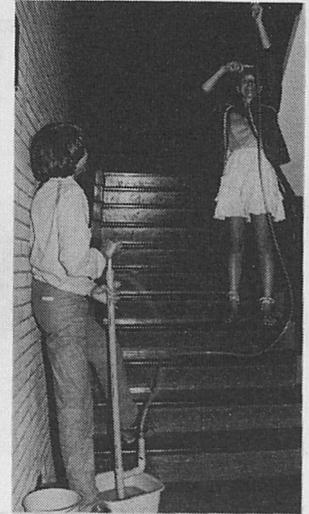
Determining the maximum height to which water can be raised in 'Working with Water'.
